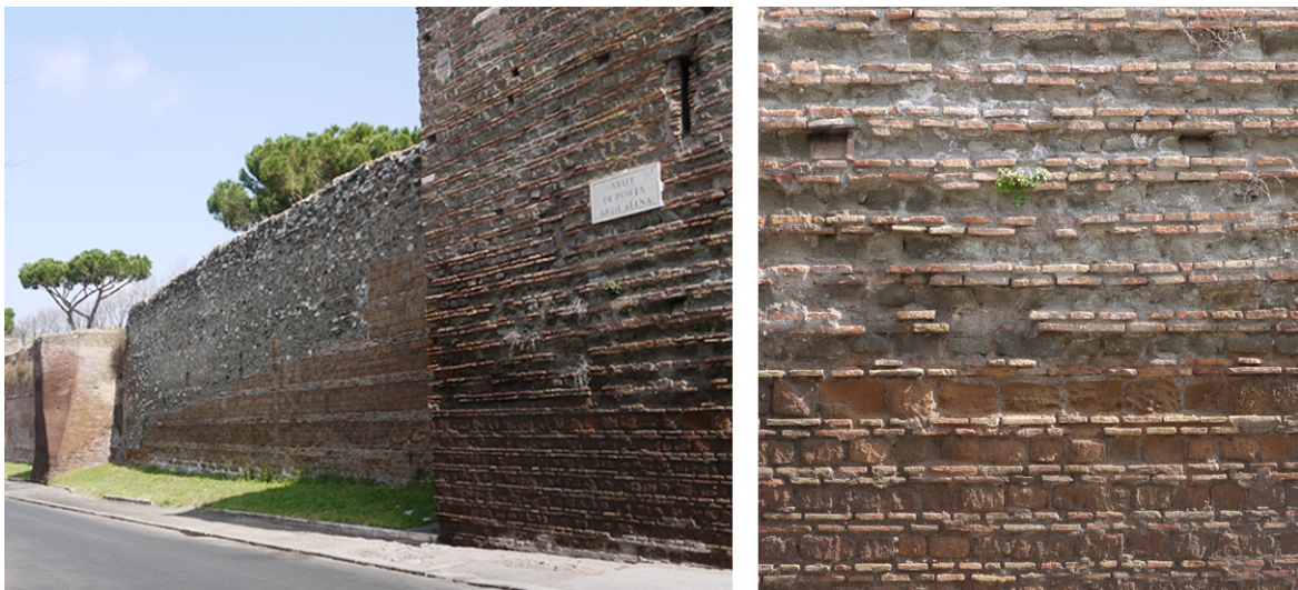
Figure 5. Banded brick and stone construction (Opus Vittatum) on the Aurelian Walls near Porta Ardeatina, Rome, 3rd Century AD. (Photograph: Ashley Paine, 2012). Figure 6. Detail. (Photograph: Ashley Paine, 2012).
