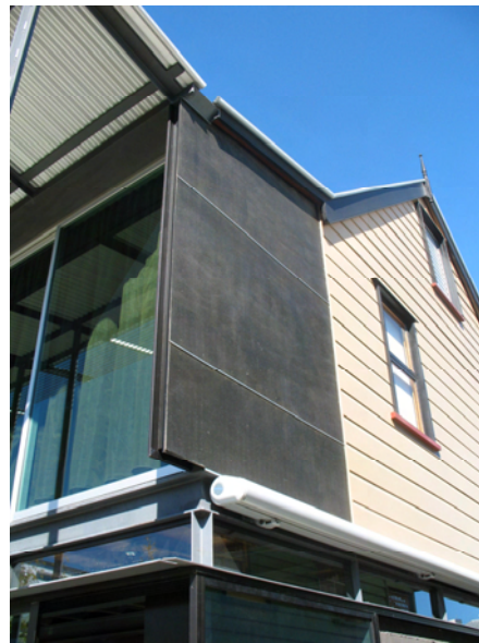
Figure 2.4 - Plywood in place of existing chamferboards to rear verandah
